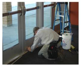
Sealing the gaps, cracks and holes throughout the building to eliminate air leakage losses is called air leakage control (ALC). Air leakage control is the first priority in any building envelope retrofit, and the primary scope of this project was to seal off 2 square feet of roof/wall joints from leaking cold air in or warm air out, utilizing a 2-part foam. Exterior doors were determined to require weather stripping and to be sealed with door sealing foam tape and sweeps.
