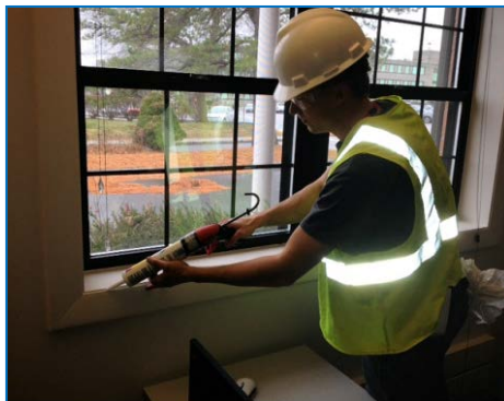
Caulk along a window sill
